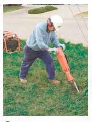
3 Drive the anchor to the proper depth, adding sections of drive steel as needed.
