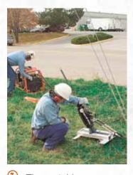
The portable power source operates the Anchor Load Locker which grips and pulls up on the adapter setting bar, rotating the anchor underground into the load lock position. The desired holding capacity is registered by the gauge on the Anchor Load Locker.
