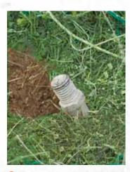
The end of the anchor rod is ground level; or in looser soils, it may be countersunk up to 12" below the surface to obtain greater holding capacity.
