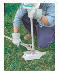
Thread a standard anchor rod into the threaded shackle of the Manta Ray anchor.
