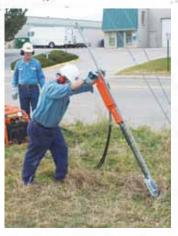
Insert drive steel into the anchor. Position at the proper location and angle.
