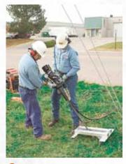
The adapter setting bar is threaded onto the end of the anchor rod. The lightweight Anchor Load Locker base and hydraulic ram system are then put in place over the adapter setting bar.
